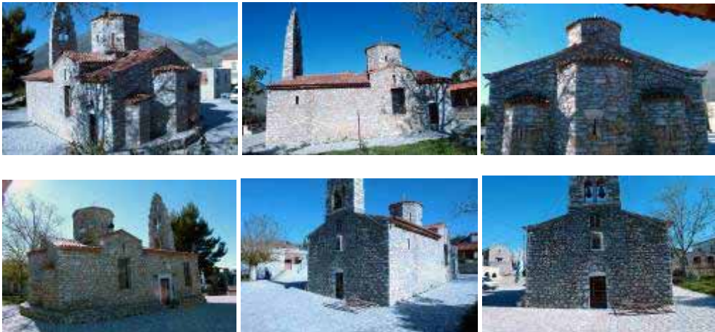
Figure 9. The photogrammetric processing was carried out rather easily using a bundle of images covering all around the entire buildings – here shown for Agios Nikolaos
